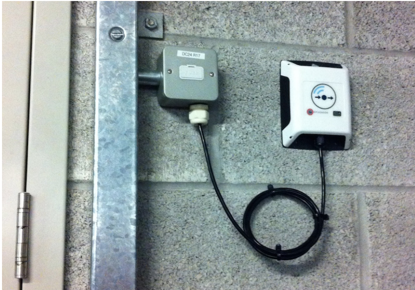
EpiSensor Range Extender, used to boost the wireless signal strength
