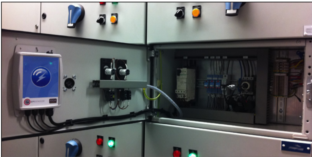
EpiSensor meter installed in an electrical distribution board
