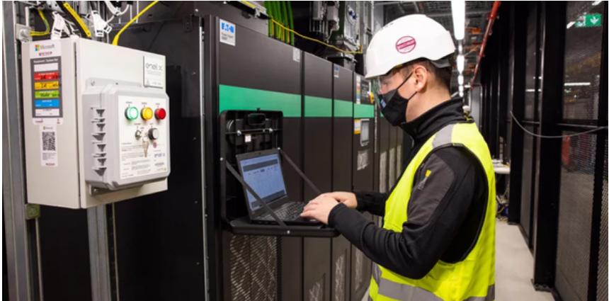
John Byrne, head of operations for Enel X UK & Ireland, performs a system test on the grid-interactive UPS inside a Microsoft datacenter in Dublin, Ireland. Photo by Naoise Culhane.
